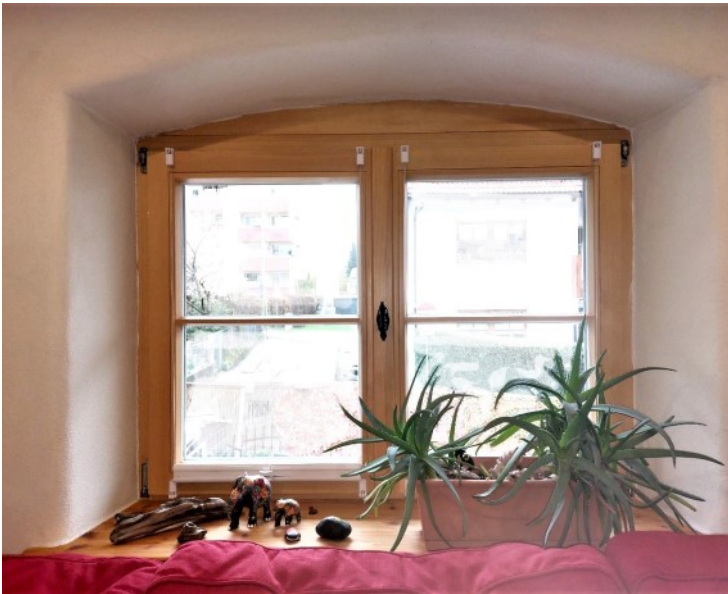
© (D. Becker) Ansprechend sanierte Fenster
